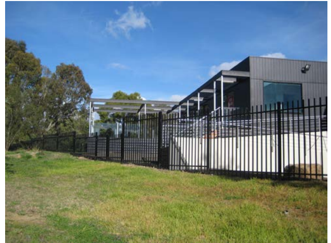
Permeable fencing with the development facing the Darebin Creek Shared Trail allows for passive surveillance
