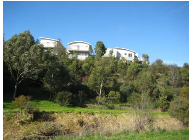
Development of buildings high on the Darebin Creek escarpment are difficult to screen.
